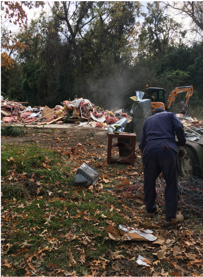
Demolition day at the old lab.
