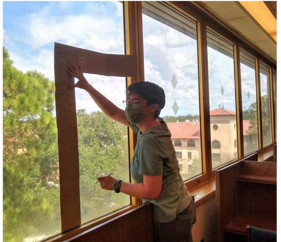
Jordan Mouton uses a template to align decals on the fourth floor of the library. The decals on the windows to her right are designed to make a reflective glow visible to birds that would otherwise would not perceive the windows. Photo by Phil Stouffer
