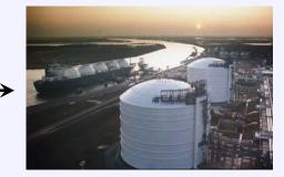
**Regasification and Delivery:** LNG is pumped from the ship to insulated storage tanks at a specially designed terminal. It is then fed into a regasification plant to return the LNG to a gaseous state. The LNG is warmed by passing it through heated pipes and various terminal components. The vaporized gas is then regulated for pressure and enters the pipeline system to be transported to end users.
