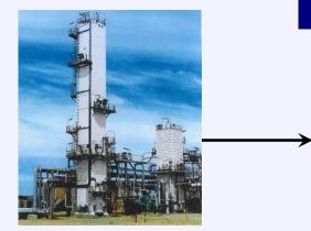
**Liquefaction:** Gas from the production field comes to the liquefaction plant. Contaminants are removed and the gas is cooled to a temperature of -256°F. By liquefying the gas, its volume is reduced by a factor of 600.
