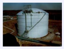
**Storage:** LNG is stored in doublewalled, insulated tanks at atmospheric pressure. These tanks are designed to prevent any leaks. There is also a dike around the wall that is capable of containing the entire volume of the tank in the unlikely event of a spill.
