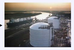
Regasification and Delivery: LNG is pumped from the ship to insulated storage tanks at a specially designed terminal. It is then fed into a regasification plant to return the LNG to a gaseous state. The LNG is warmed by passing it through heated pipes and various terminal components. The vaporized gas is then regulated for pressure and enters the pipeline system to be transported to end users.
