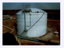
Storage: LNG is stored in double-walled, insulated tanks at atmospheric pressure. These tanks are designed to prevent any leaks. There is also a dike around the wall that is capable of containing the entire volume of the tank in the unlikely event of a spill.
